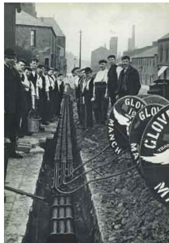
Laying the first electricity networks in Ancoats.
