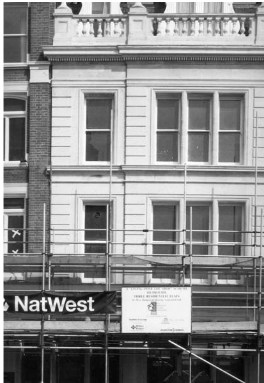
EXHIBIT 36: West Hampstead Housing Association is a pioneer of living over the shop. On Kilburn High Road they have undertaken 15 projects, housing several hundred people. Using commercial leases that enable the owner to regain empty possession, the association has converted and repaired the interior, while the property owner is responsible for external work.
