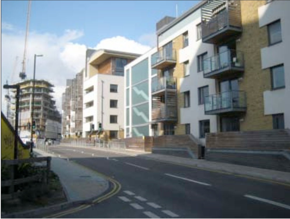
The back of the supermarket on the new road
