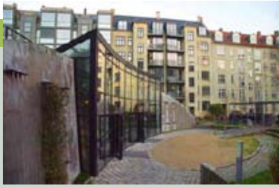
1990's Hebedygarde, Copenhagen Pioneering test-bed for turn of the century apartment blocks.
