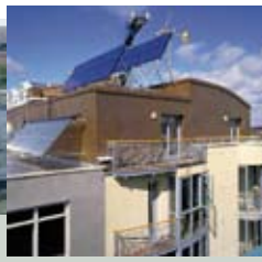
1994 'Green building', Dublin Demonstration low energy block in Temple Bar with solar and wind power and ground source heating.
