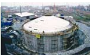
1996 Friedrichshafen, Germany Large-scale scheme which meets all its heating from interseasonal solar thermal storage.
