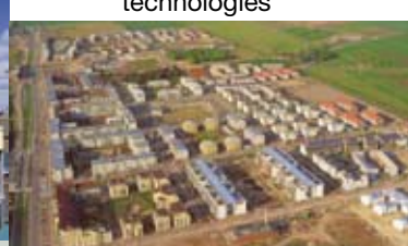
2000- SIBART network Large-scale (2000+) new urban extensions in Germany, Netherlands, Sweden, Finland and the UK with low carbon energy strategies
