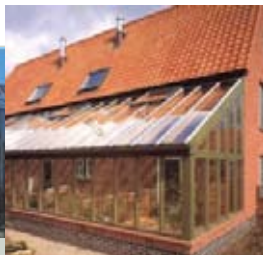
1994 Autonomous House, Nottingham Super-insulated family home which balances all its needs by generating solar heat and power
