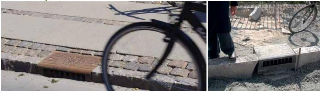
Figure 12, 13 - Rainwater gullies built into the curb to create a smoother, more bikeable path (illustrations from Copenhagen City of Cyclists Bicycle Account 2010 pg 66)
