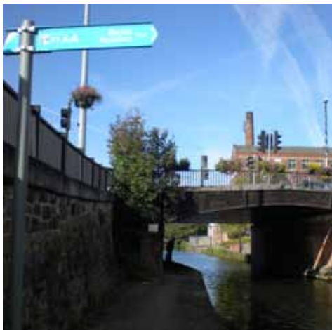
View to Patricroft Bridge from Bridgewater Canal
