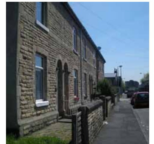
Terraces on George Street
