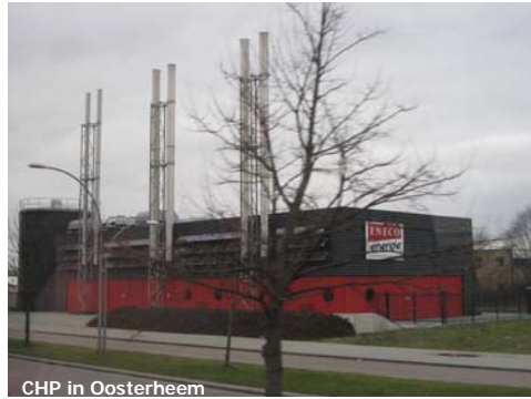
CHP in Oosterheem
