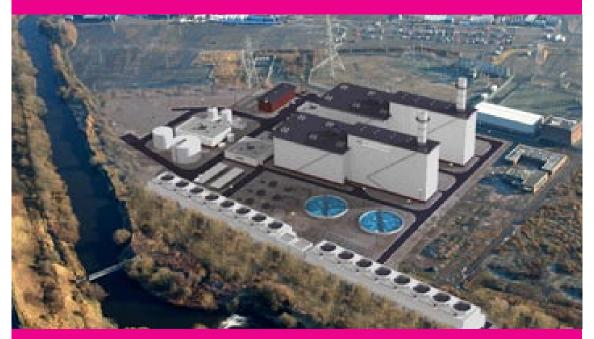
Concept plan for heat offtake from Carrington power station: A concept plan and strategy for using waste heat from the proposed gas fired power stations at Carrington, with the potential to supply a corridor extending all the way to Manchester City Centre. It would be one of the largest single carbon reduction measures in Greater Manchester.
