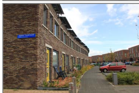
Solar panels in Almere Poort
