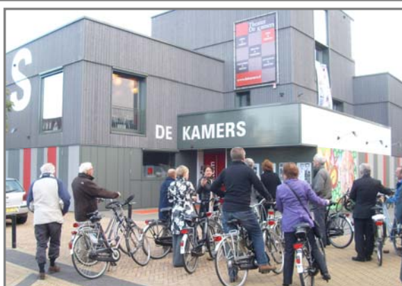
Top: Vathorst railway station Bottom: De Kamers Community Building
