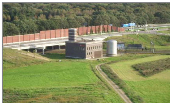
Above: Vathorst centre Below: Vathorst District Heating Station
