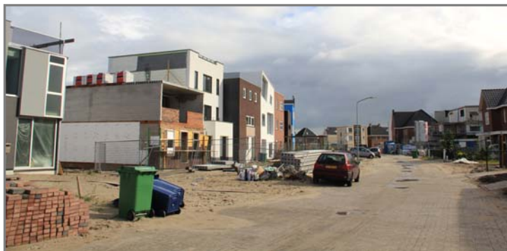
Residents are living on a building site until the development is completed
