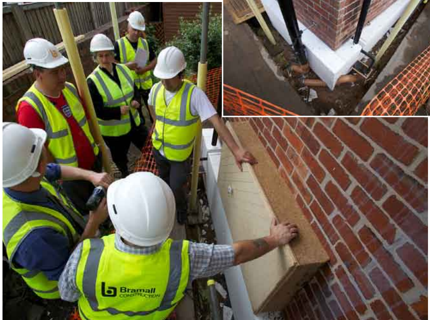
Builders debate the fixing solutions for the external insulation system.
