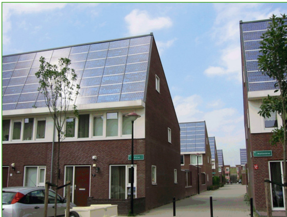
Above: 500 dwellings in Nieuwland, Amersfoort were provided with a photovoltaic system, with a total project size of 1 MWp
