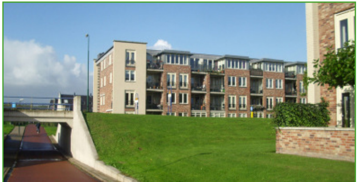
Cycle underpass in Houten
