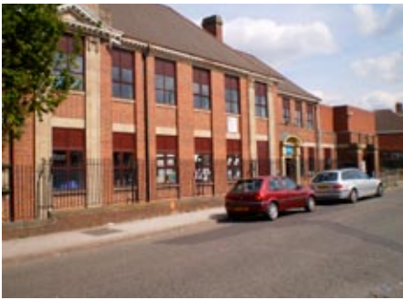
Kings Hill primary school, Old Park Road
