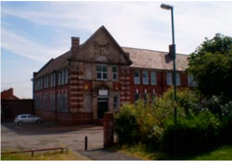
The Innovation Works @ Rubery Owen, Booth Street
