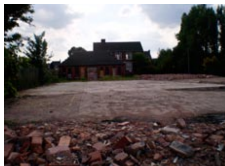
Half demolished leisure centre, Victoria Road
