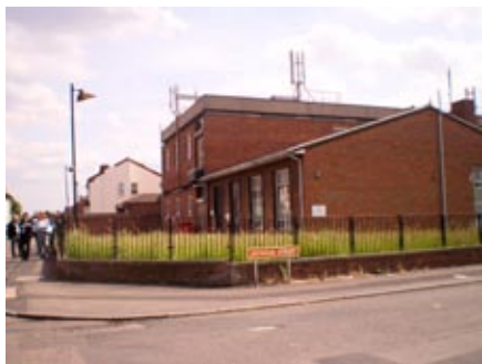
Vacant BT Exchange, Old Park Road
