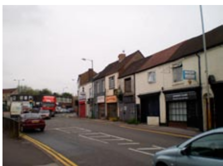
Pinfold Street and the derelict shop units
