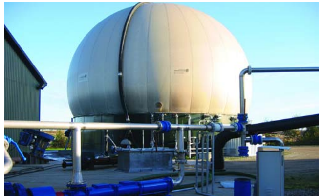
D.12 Hashøj biogas storage tank
