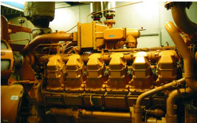
D.11 Hashøj biogas CHP engine
