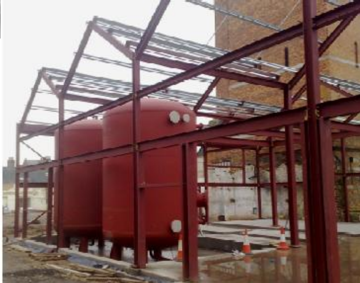
Thermal stores being installed
