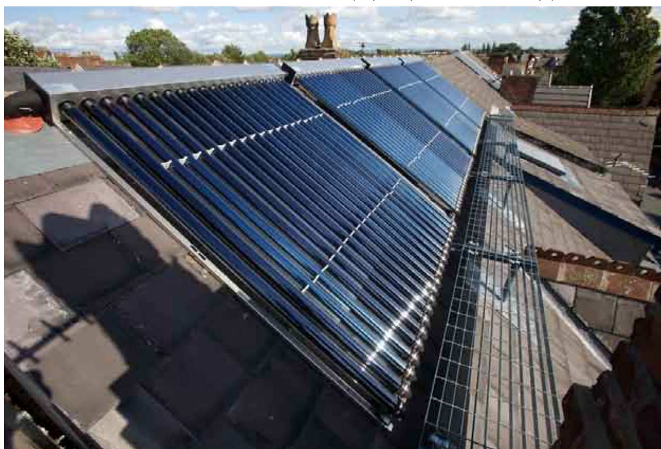
^ A retro-fitted Victorian semi-detached in Manchester - external wall insulation, new roof insulation and solar thermal hot water tube. For more detail see ( http://superhome.urbed.coop/ )
