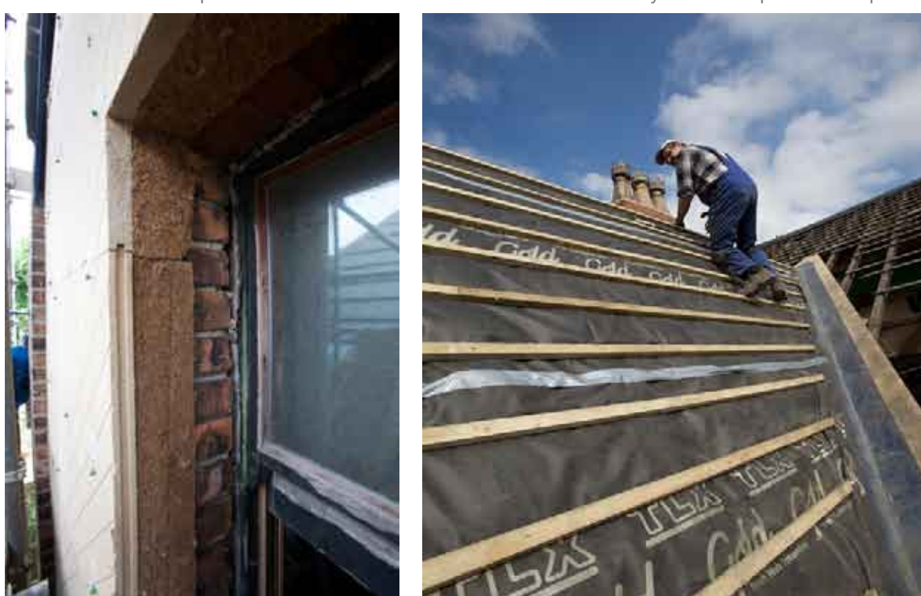
^ A retro-fitted Victorian semi-detached in Manchester - external wall insulation, new roof insulation and solar thermal hot water tube. For more detail see ( http://superhome.urbed.coop/ )
