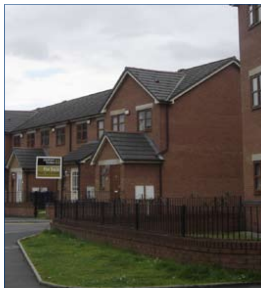
Left: new built terraces on Baron Street
