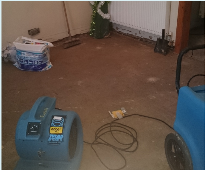
Drying out was by electric heaters and dehumidifiers.
