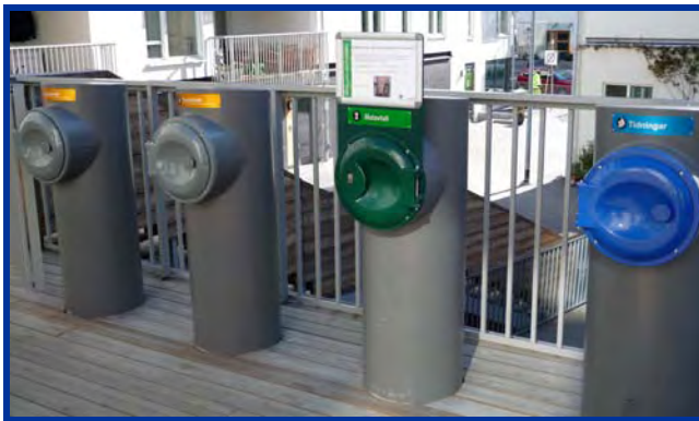
Figure 17: Envac recycling system, Hammarby, Stockholm
