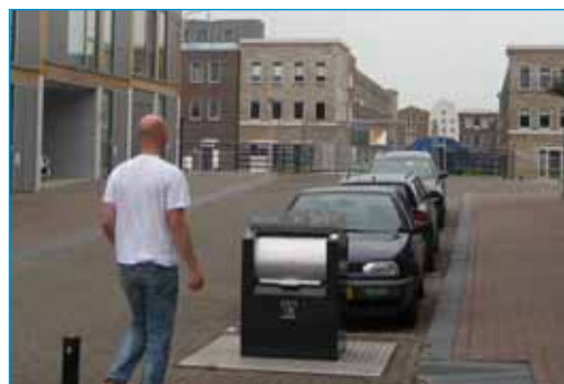
Underground waster storage
