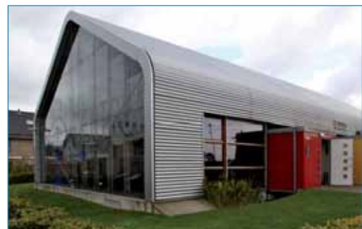
Vathorst Information Centre, a dedicated facility for visitors and residents and includes a café and scheme model
